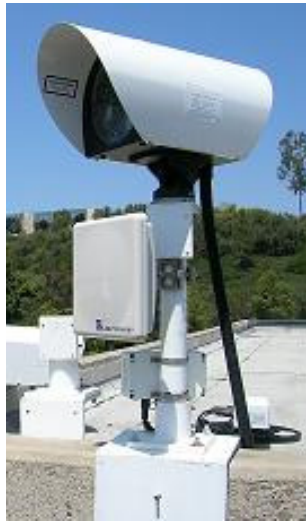
Figure 2-1: Typical DualPath Optical Wireless + RF Mount Installation
